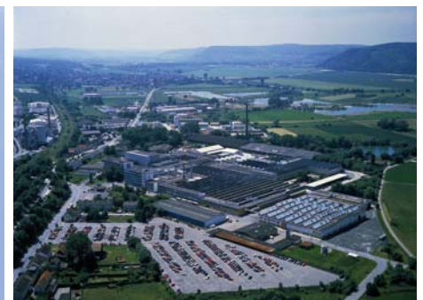
Stiebel Eltron plant in Holzminden, Germany
