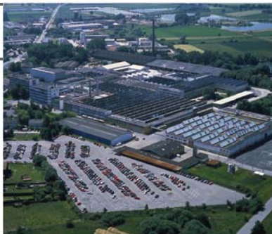
Stiebel Eltron's plant in Holzminden, Germany.
