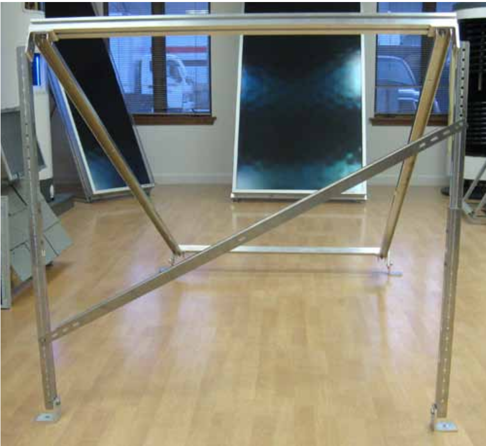
Step 30: Install one of the cross braces using two 1/4" nuts, bolts and washers.
