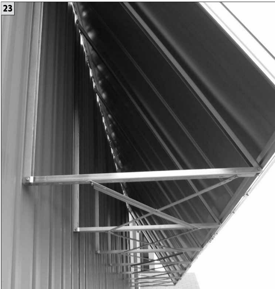
Figure 23: Typical wall-mount installation of a 60° collector array.
