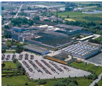
Stiebel Eltron's plant in Holzminden, Germany.
