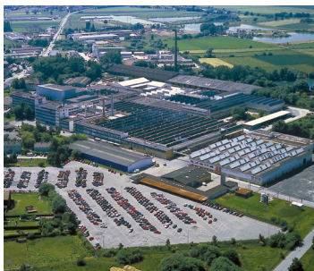
Stiebel Eltron's plant in Holzminden, Germany.
