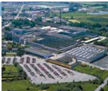
Stiebel Eltron's plant in Holzminden, Germany.
